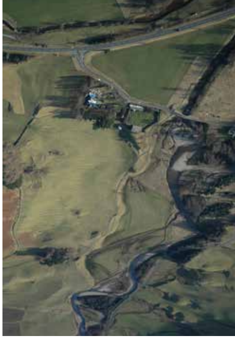
Above: To the north of Bridge of Cally, a section of the military road built under the supervision of Major William Caulfeild in the mid-1700s AD is visible. The distinctive banks of earth and stone that were thrown up along either side of the road by the soldiers during its construction are particularly clear, photo © Perth & Kinross Heritage Trust Left: Major Caulfeild's Bridge over the Shee Water at Spittal of Glenshee. In the field to the right of the present church, the rectangular outline of the 18th-century chapel, contemporary with the bridge, can be observed. The long lines of rig and furrow cultivation can also be appreciated within the same field in this image, photo © Perth & Kinross Heritage Trust
