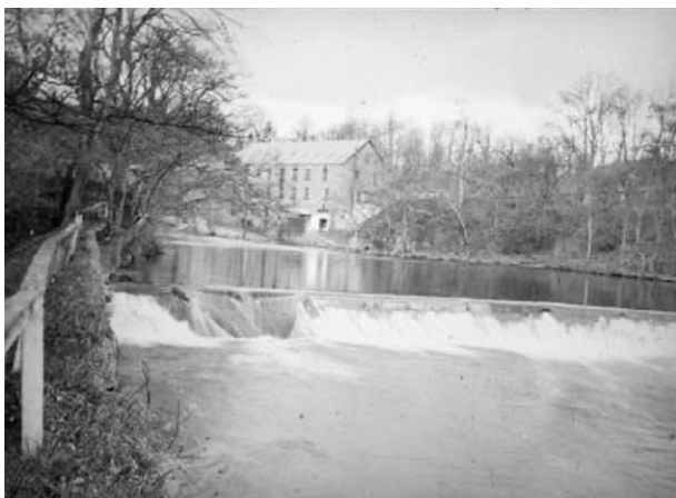
Oakbank weir, a modest 1.5m high weir. Bramblebank is in the background, the still-water formed by Oakbank's weir almost affecting Bramblebank
